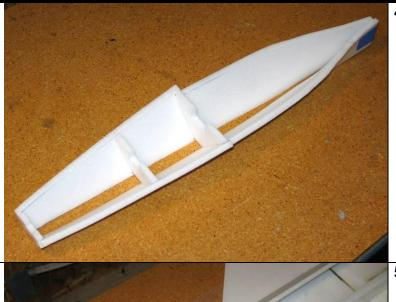
**4.** Glue the bottom half of the three fuselage bulkheads (the ones with the notch on top) to one of the lower forward fuselage sides at the locations shown on the plans, making sure they are perpendicular. Then set the fuselage sides upright and flat on the workbench, apply glue to the edges of the bulkheads, and then glue the two fuselage sides together.
