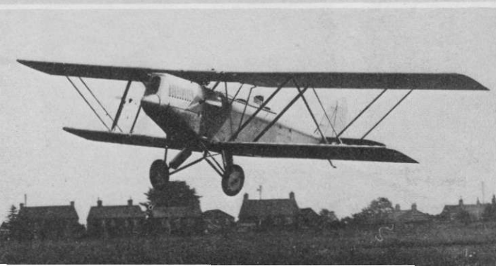
Early photographs of Parnall Elf show distinctive Warren girder wing bracing in head-on flying shot above. Full length top wing ailerons clearly visible at right, with full length hinge on lower wing to permit wings to swing back for storage. Left: fin and rudder hinge line differs from restored machine at Shuttleworth. "Air Portraits" & "Flight" photos.
